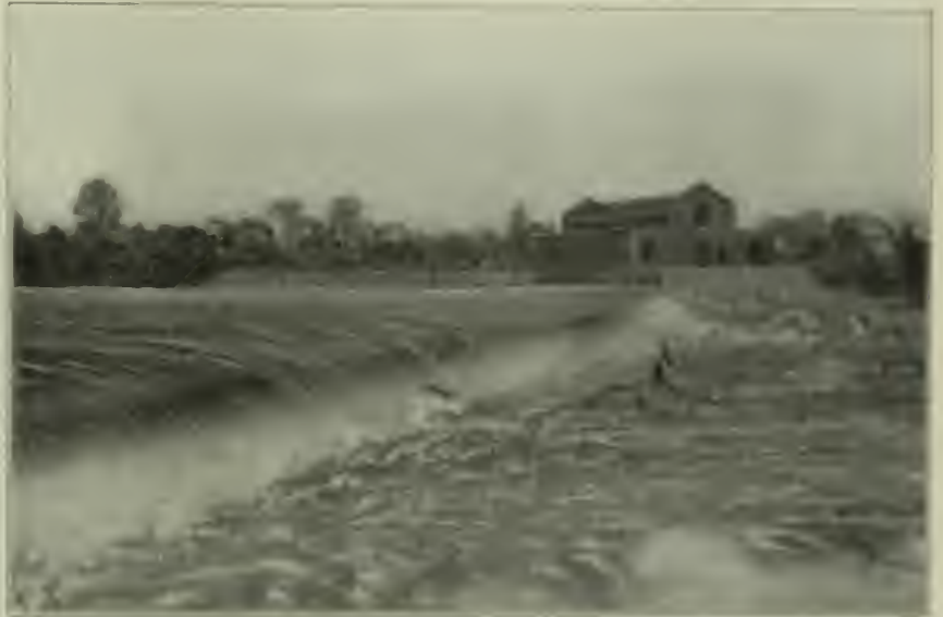
FIG. 1. THE DAM AND TURBINE HOUSE AT MILFORD.
